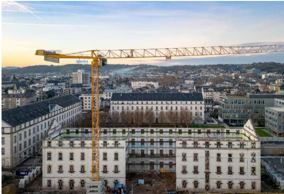
Rehabilitation of the Caserne Brune in Brive la Gaillarde - Kalilog -136 units
