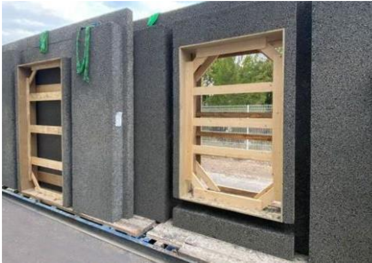
Prefabricated wooden concrete facades.
